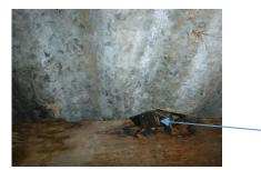
Moisture present at the base of the shower recess indicative of current leakage
