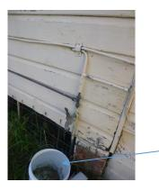
The NW exterior tap was dripping at the time of the inspection
