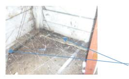
Extensive wood decay damage present to bottom wall plates at the southern and western sides of the garage
