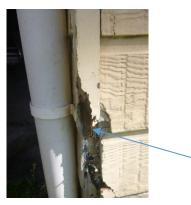
Moderate wood decay damage to the corner cladding battens – southern corner of the kitchen pictured
