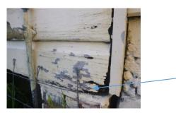
Moderate wood decay damage present to the ends of the cladding at the western corner of the bathroom
