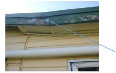
Moderate wood decay damage to the barge boards at the western corner of the house
